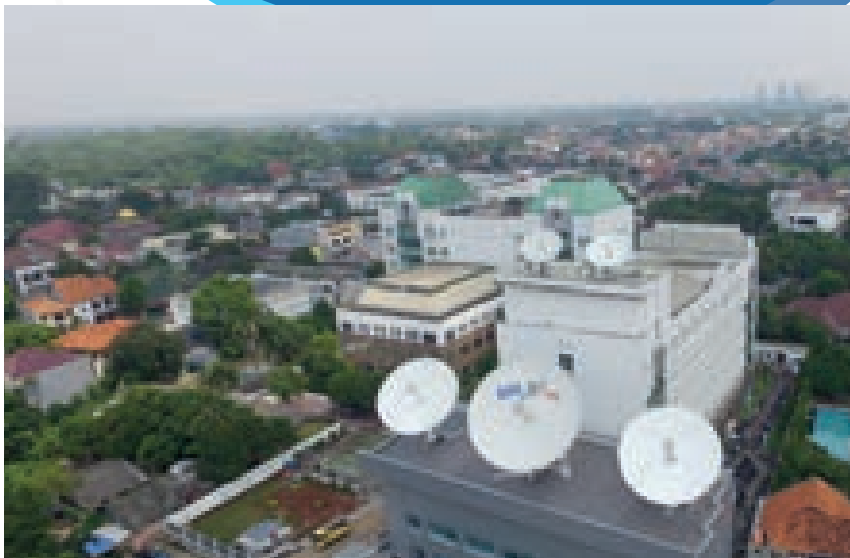
BRIsat Control Center
